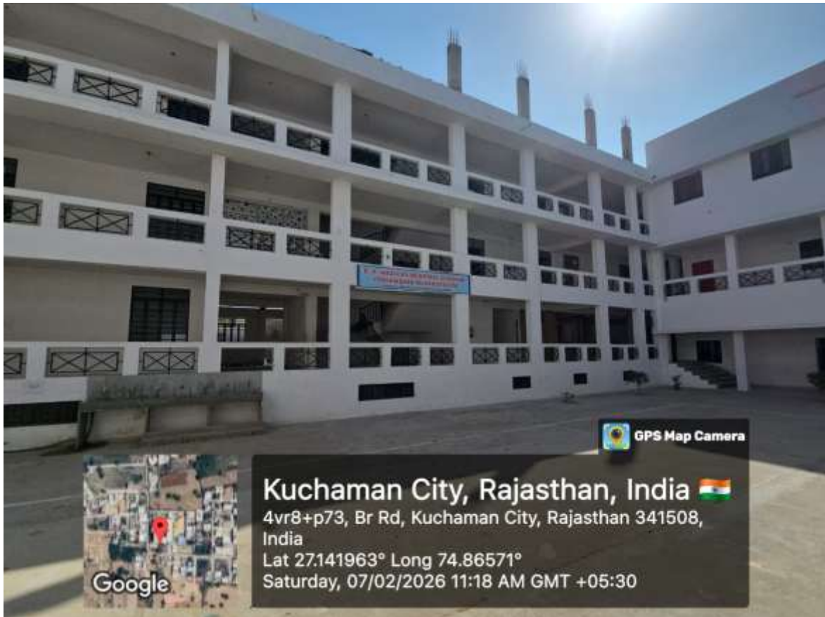
Building Rear View
